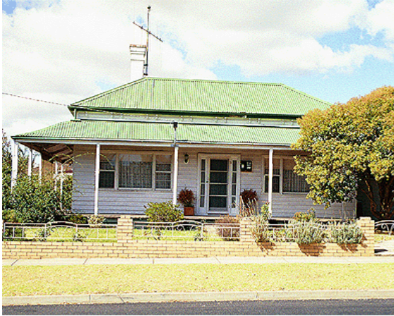
FIG. 16. 11 Guild Street (windows, verandah posts and decoration and fence appear to have been changed c1950s.)
