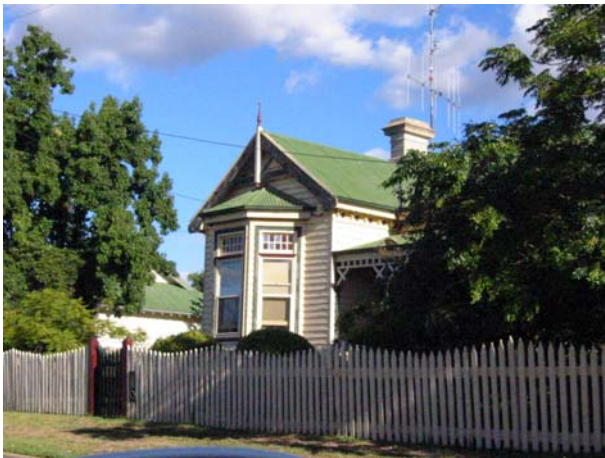
FIG. 3. House at 36 Park St Lot 115.
