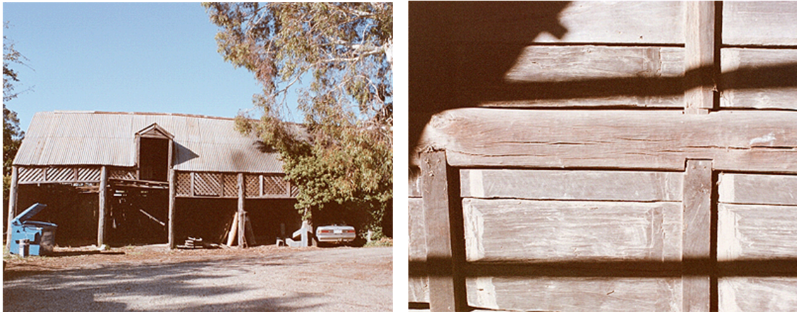
FIG 8 Royal Hotel Stables and construction detail on the right.
