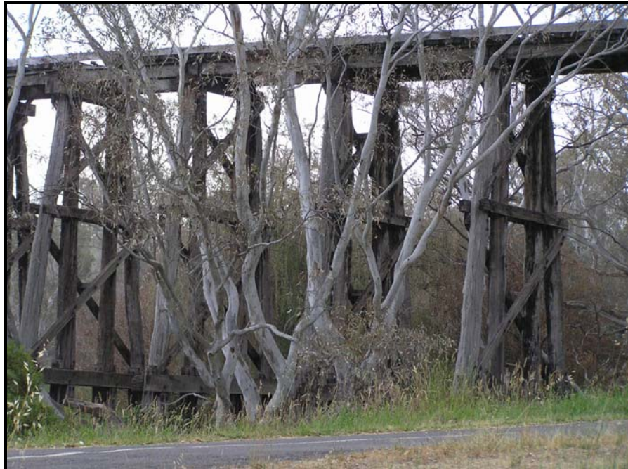
Timber trestle bridge in the Pyalong Rural Town Heritage Precinct.
