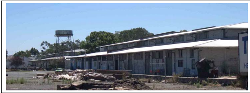
Fig. 8. Mobilisation storage sheds. Source: Lorraine Huddle Pty Ltd.
