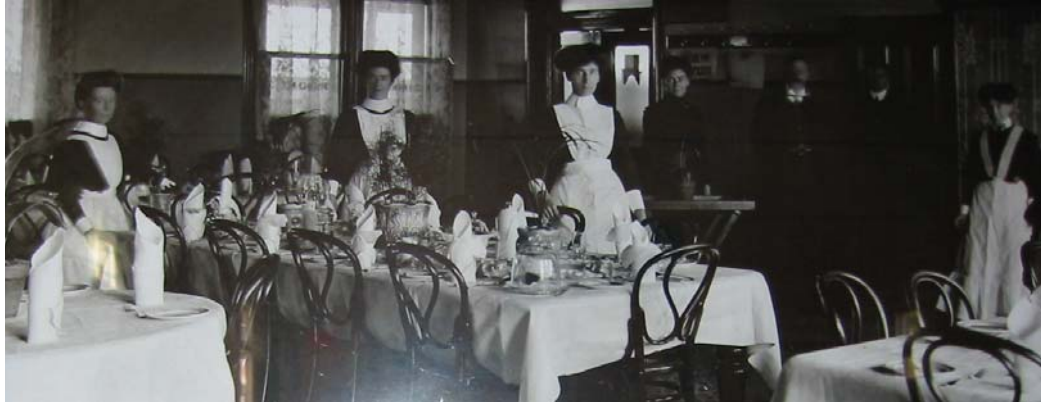
Fig 3. Tallarook Railway Station Refreshment Rooms. 1926. Source: Tallarook Mechanics Institute.
