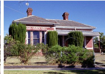
Fig 35 62 High Street Victorian Italianate. Source: Lorraine Huddle 2002
