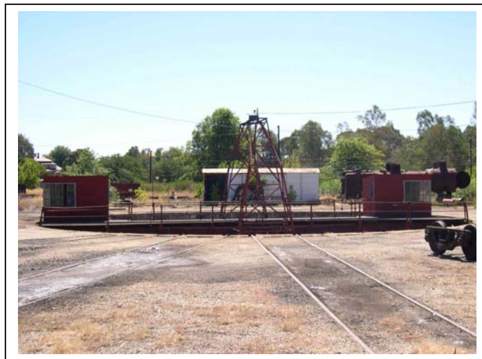
Fig. 5. Turntable infrastructure. Source: Lorraine Huddle Pty Ltd.
