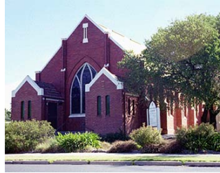
Fig 28 Uniting church (1925) (formerly Methodist) is designed in a rather conservative Interwar Gothic style. Source. Lorraine Huddle 2003
