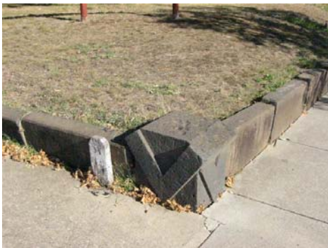
FIG. 48. Retaining wall made from recycled bluestone. Source: Lorraine Huddle 2003.
