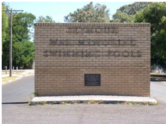
Fig.9. Entry to Memorial Swimming Pools. Source: Lorraine Huddle Pty Ltd.
