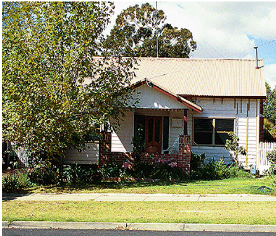
FIG. 15. 7 Guild Street. (windows altered and the fence removed.)
