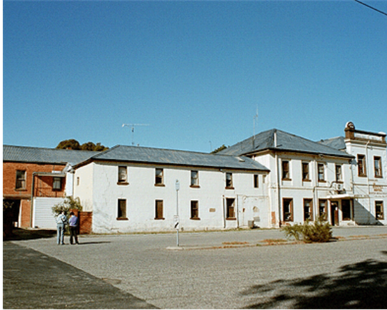
Fig. 6. Royal Hotel showing the various stages of development. Source: Lorraine Huddle Pty Ltd 2002
