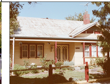
Fig 40 84 High Street. c1925 Californian Bungalow. Source: Lorraine Huddle
