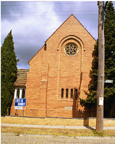
FIG. 24. St Andrew's Presbyterian Church and Hall.
