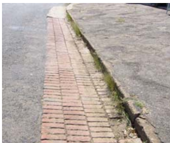
Figs. 10 and 11 showing the four deep red brick tray gutter near the hotel with a more recent kerb in concrete. The detail on the right shows the red brick gutter as a 3 deep spoon drain.
