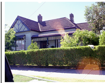
Fig 36 14 Butler Street. c1905 Federation Arts and Crafts residence. Source: Lorraine Huddle 2002
