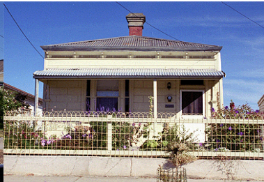
Fig 34 82 High Street Victorian Italianate Source: Lorraine Huddle 2002
