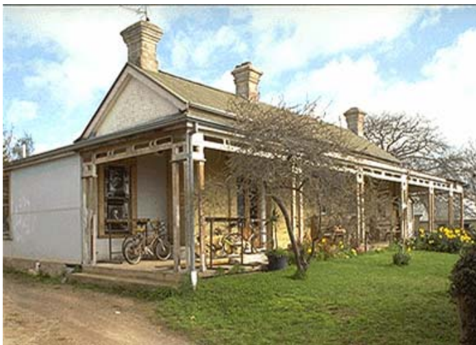
FIG 10. 3-5 Chapel Street Source: Lorraine Huddle Pty Ltd 2002 Built as a double fronted house with English bond face brickwork, ruled stucco facade and a timber verandah. It was extended to the south, in a sympathetic style to create a second entrance with double doors placed between pronounced pilasters. The return verandah has duplex
