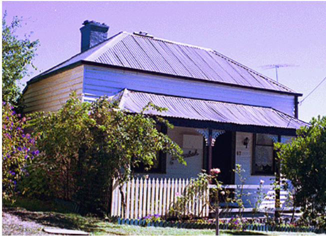
FIG. 21 “Moombah” House, 67 Fitzroy Street (DB 260)
