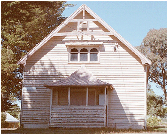
FIG 15. Gavan Hall, built c1904 is a large timber gabled building with a corrugated iron roof with decorative roof vents with delicate concave front porch, and Federation Carpenter gothic style architectural detailing, such as the flying gable end with finial, in a picturesque treed setting of Cypress and Spruce trees. Source: Lorraine Huddle Pty Ltd 2002.
