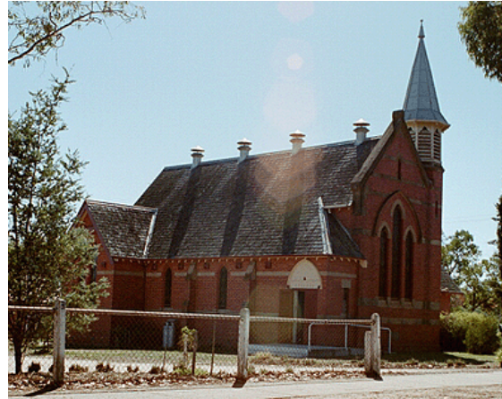
FIG 16 St George's Presbyterian Church. Federation Gothic. Source: Lorraine Huddle Pty Ltd 2002.
