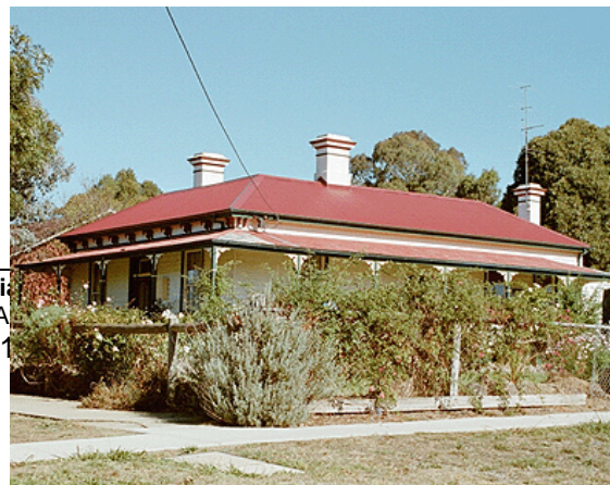
FIG. 12. Former Presbyterian Manse 26 Hamilton Street, 2002. A substantial Victorian weatherboard house with hipped M roof clad in painted galvanised corrugated iron and decorative chimneys. The return skillion
