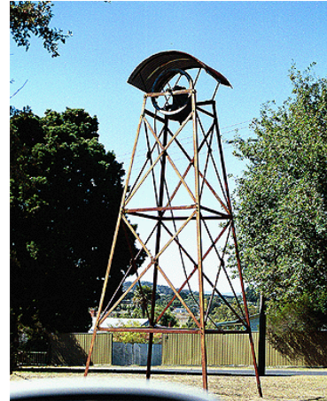
Fig. 10. Angled iron framed bell tower.
