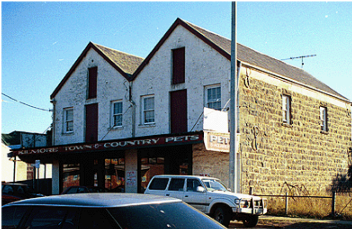
FIG 15 Former Hudson Warehouse. Source: Lorraine Huddle Pty Ltd.
