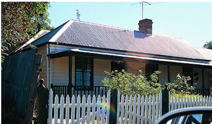
FIG 11 9 Chapel Street. 2002 Source: Lorraine Huddle Pty Ltd
