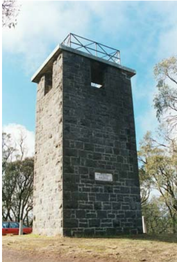
FIG. 21. View of the tower with plaque. Source: Susie Zada 2003.
