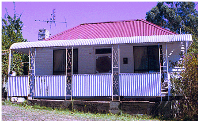
FIG 20 House, 65 Fitzroy Street (DB 998)
