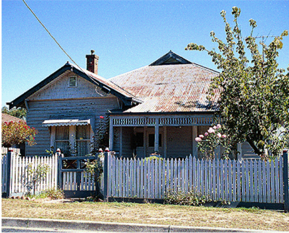
FIG 9. House, 53 Albert Street 2002 (DB 997)
