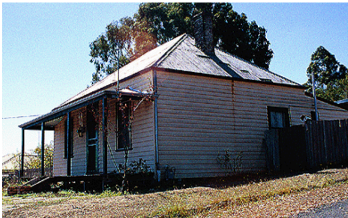
FIG 10. House, 58 Albert Street 2002 (DB 423)
