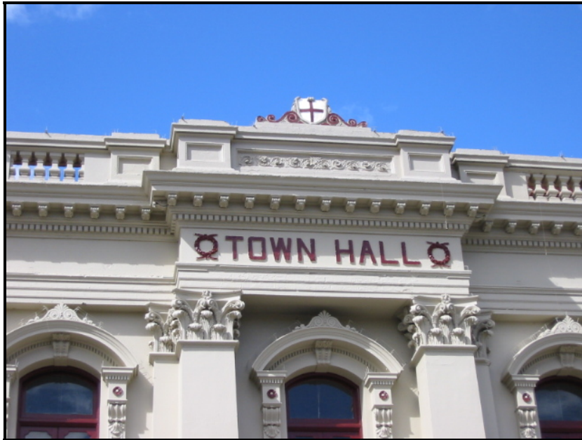
Kilmore Town Hall (Café) in the Kilmore Town Centre Heritage Precinct.
