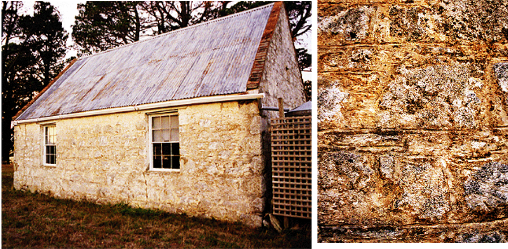
FIGS. 10, 11 Emu Flat Uniting Church showing granite stone wall construction. 2002
