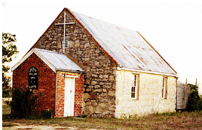
FIG 16. Emu Flat Uniting Church 2002, showing the granite stone walls of the main room and c1898 red brick porch. FIG 17 (below) Interior of the church 2002.
