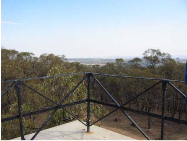
FIG. 22. View of concrete top, deteriorating black paint on metal balustrade and view to the Kilmore Gap. Source: Lorraine Huddle 2003.
