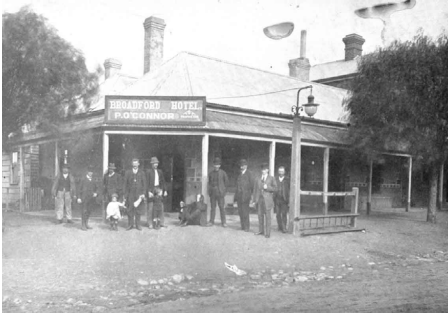
FIG. 13. : Broadford Hotel, P. O'Connor Proprietor. Note the brick and stone construction with quoins around the window and door openings, the two storey building to the right, and the timber 'masonry' building on the left. These may all be various parts of the hotel.
