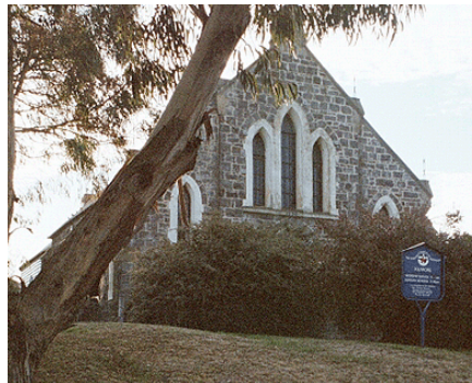
Fig 36. Former Wesleyan Methodist Church at Kilmore Source: Lorraine Huddle 2002.
