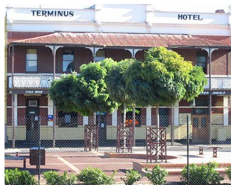
Fig 24. Terminus Hotel at Seymour Source: Lorraine Huddle 2002.
