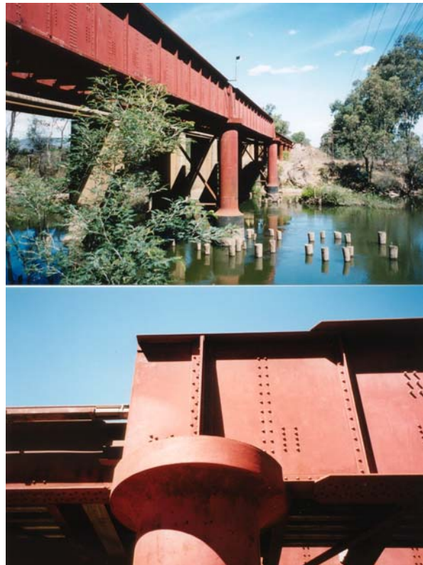
Riveted Iron Plate Web Girder Railway Bridge 1872, Seymour Source: John Jennings.
