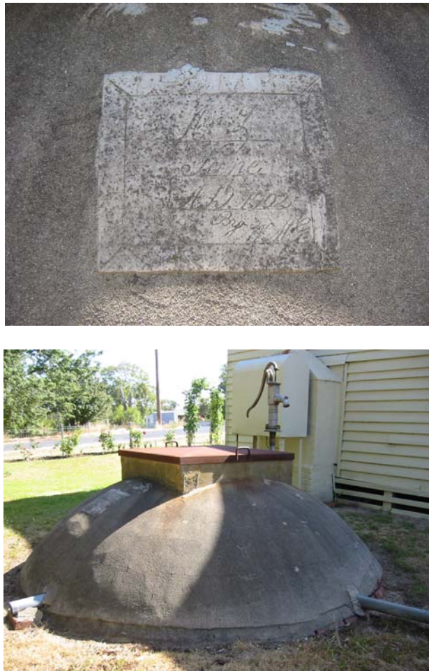
Fig 5. Top: Detail of the 1902 inscription by the local builder, Zoch, on the underground water tank in Pyalong. Bottom: View of the domed top and hand pump
