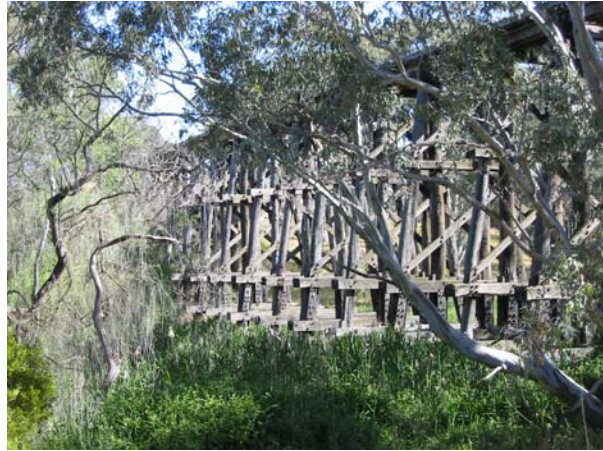
Timber Trestle Railway Bridge, Pyalong Source: Lorraine Huddle Pty Ltd.
