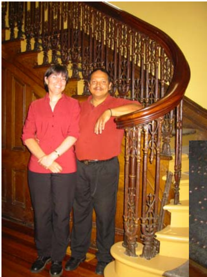
Fig 4 Kilmore Town Hall: Café and Restaurant proprietors, Susan and Peter Seibel, next to staircase with restored cast iron balusters, carved timber banister and lead treads with copped nail decoration. Source: Lorraine Huddle Pty Ltd.
