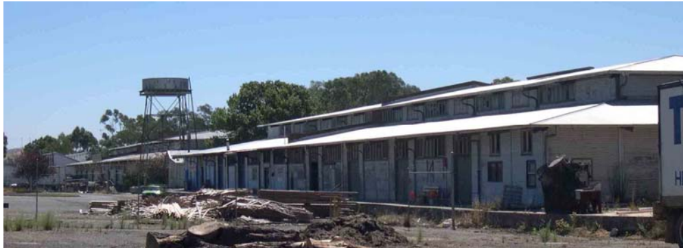
Figure 2: Storage warehouses and elevated tank Source: Lorraine Huddle Pty Ltd, 2006
