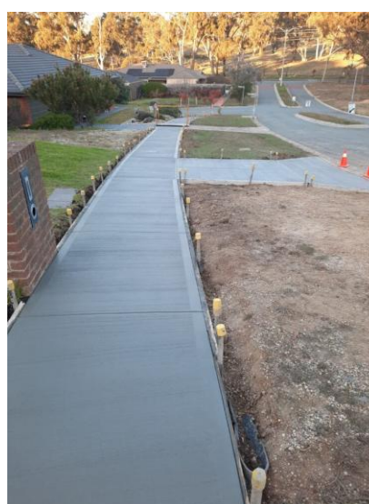
Footpath construction O'hara Drive Seymour
