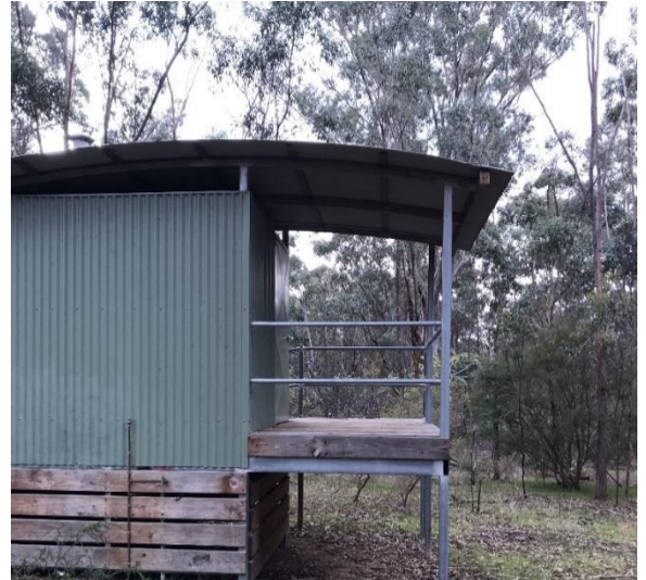
Figure 10 Existing Toilet facility
