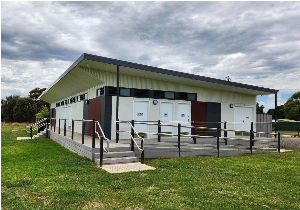
Figure 22 Wallan Secondary College pavilion
