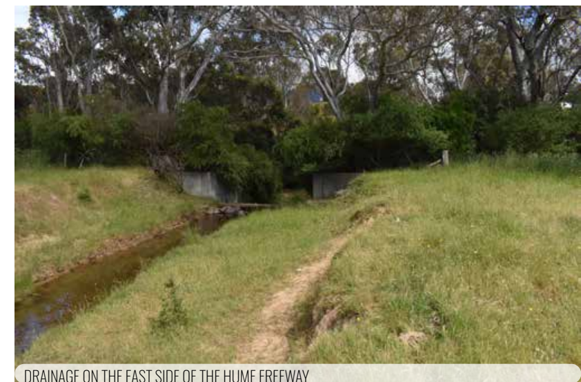
DRAINAGE ON THE EAST SIDE OF THE HUME FREEWAY
