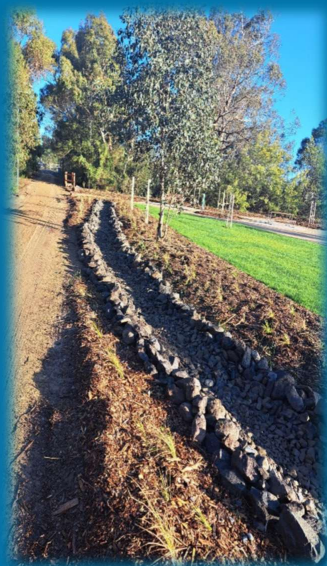
Wallan Community Park (Swale drain)
