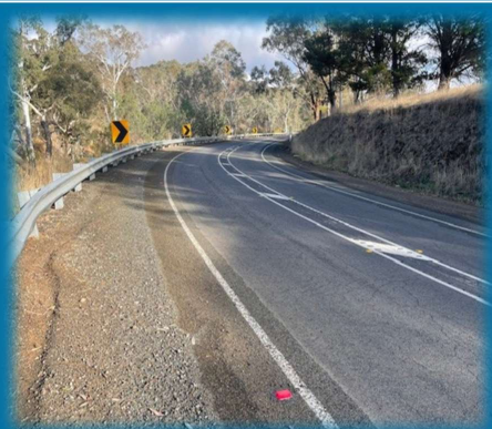
Blackspot – Seymour-Pyalong Road- Shoulder widening
