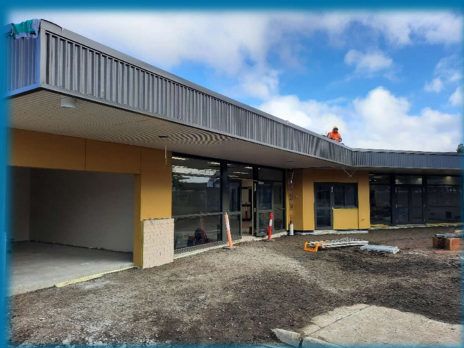
Greater Beveridge Community Centre Expansion- Exterior (Work in Progress)
